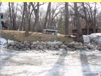
A portion of the completed Tanglefoot shoreline project
