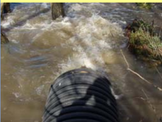
Water returning to Ventura Marsh from dredging containment site
