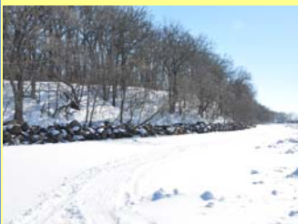
Shoreline Stabilization Project at McIntosh Woods State Park
